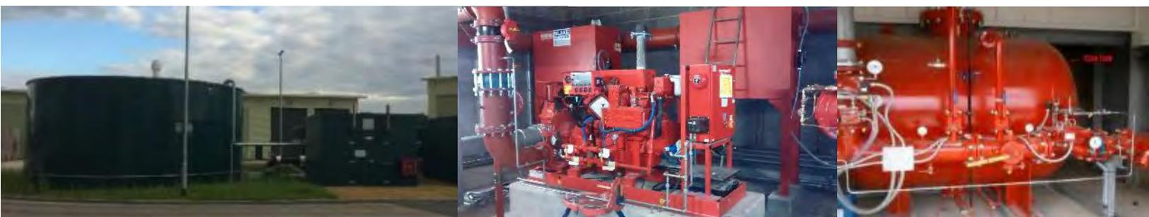
*Left to right: Fire water tanks and pump house at a recycling plant, inside a pump house, foam storage tank and systems at a large waste recovery plant*
